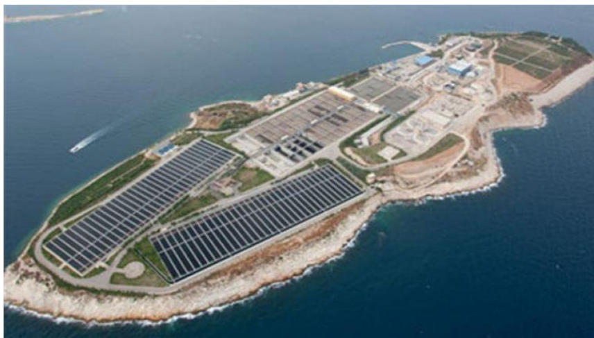
Figure 8: Aerial view of the Psyttalia WWTP
